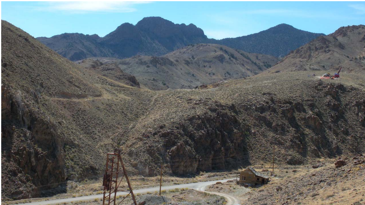
Photo 6 View of Nivloc Structure looking southwest
